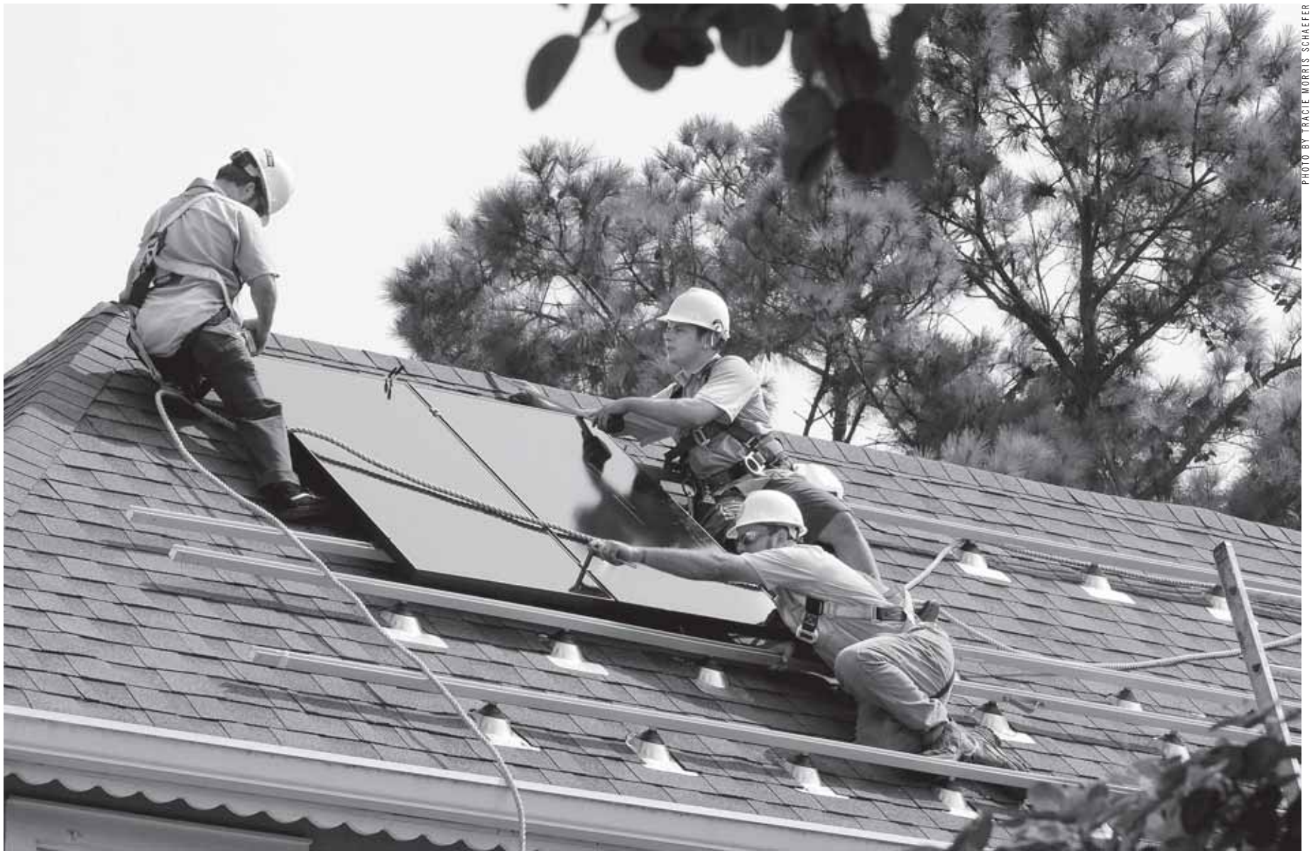
SouthCoast Solar employees, from left, Tim Coats, Micah Galy and Issac Wright, install a solar panel on a customer's roof.
